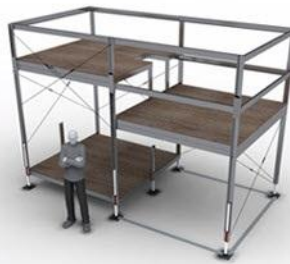
2 assemble frame and floors
