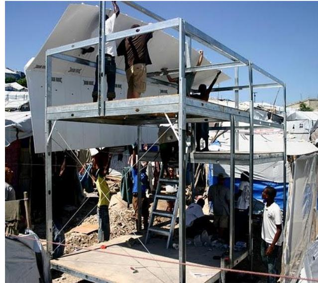
Each TShel2 when palletized is 8' x 4' x 2.5' and weighs 1200 lbs. Depending on configuration, 30 each TShel2 should ship in an ocean freight container. The material kits can be distributed locally in lighter weight bundles as needed.
