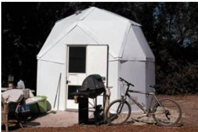
U-Dome110 at River Haven transitional shelter community, Ventura, CA
