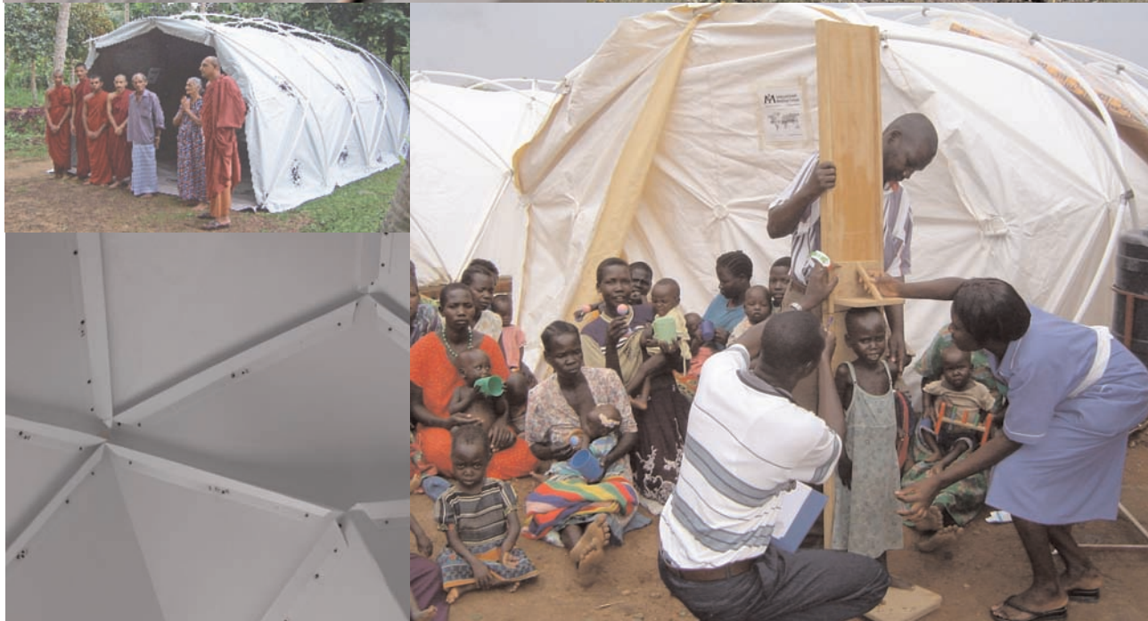
(Clockwise from upper left) 1. Q-Shelter with aluminum poles for use in cold climates. 2. U-Dome in Arcata, CA. 3. In Uganda, an International Medical Corps portable clinic in a Shelter Complete. 4. Close-up detail of internal "origami beams" made from folded flaps of the flame retardant corrugated polyethylene panels. 5. In Galle, Sri Lanka, monks at the entrance of a Shelter made with USAID supplied material.
